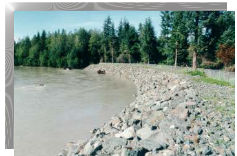
Mendenhall River revetment, Alaska
