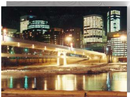
Northwest Light Rail Transit Bridge, Bow River, Calgary
