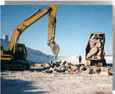
Imperial Oil Mackenzie River Artificial islands ice scour repairs, March, 1998
